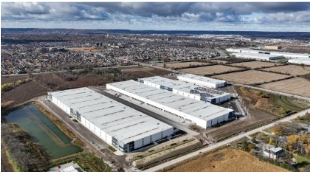
The facility in Milton, Ontario, also includes an enhanced envelope and precast panel insulation to reduce air leakage. Credit: BGO
